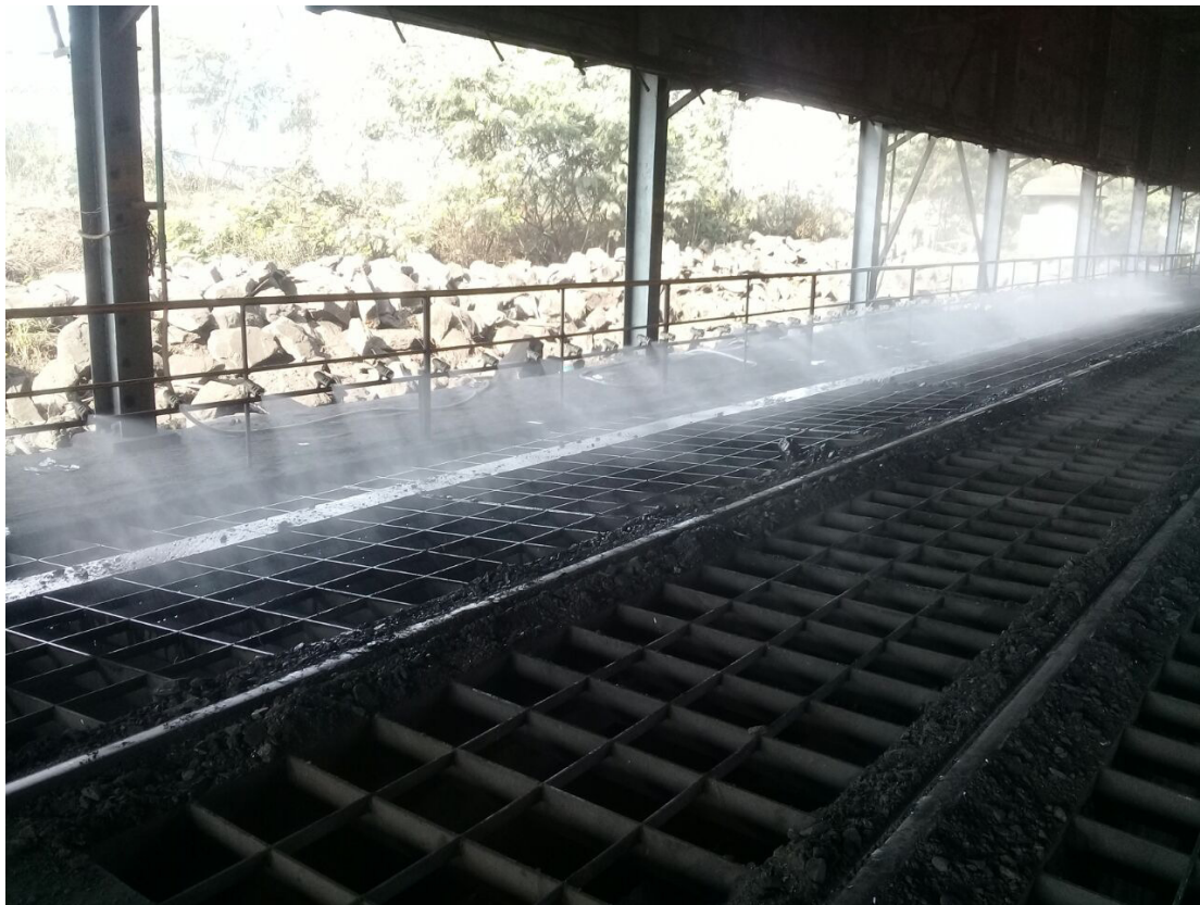
Eyeball Type misting Jet Nozzle with Housing in operation at Tracker Hopper
